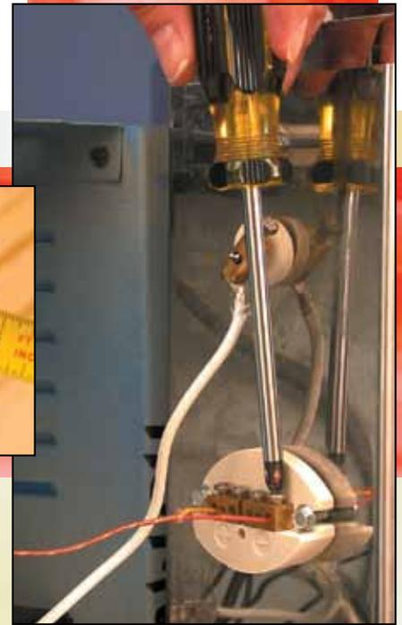
*A loose thermocouple screw can cause erratic temperature readings in the controller display window.*
